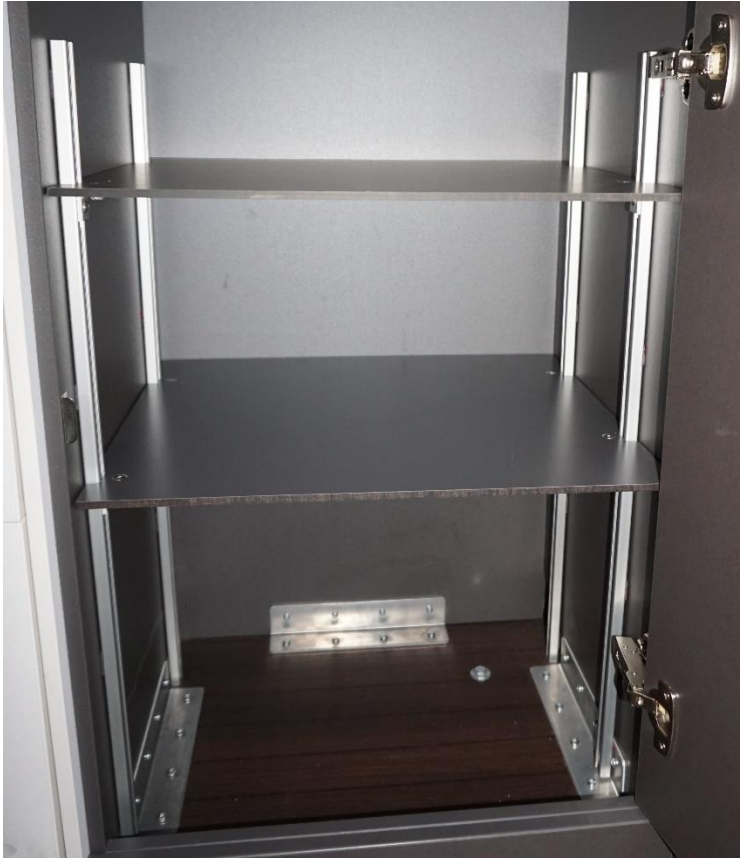
Figure 7. Positioning of aluminium tracks and shelves
