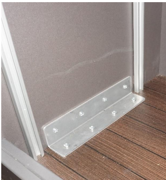
Figure 5. Positioning of aluminium track (B) left hand side.
